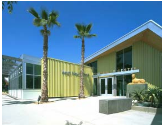
West Hollywood Community Center Hollywood, California
